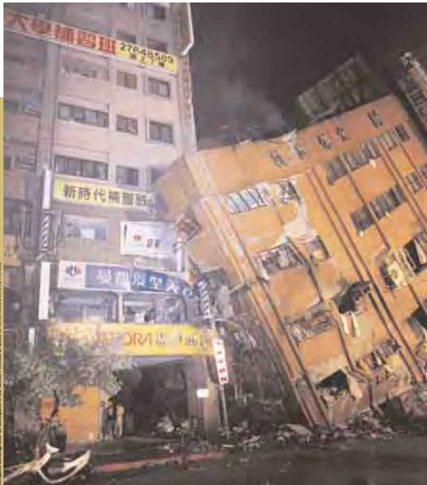
Collapsed buildings after an earthquake in the Taiwan Province of China. LO TSUNG HSEUNG/ISTOCK PICTURES
